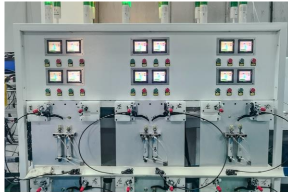
OIL LEAKAGE 100% TESTED
